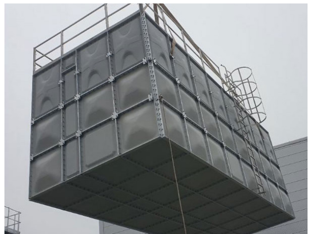
Final GRP Tank placement
